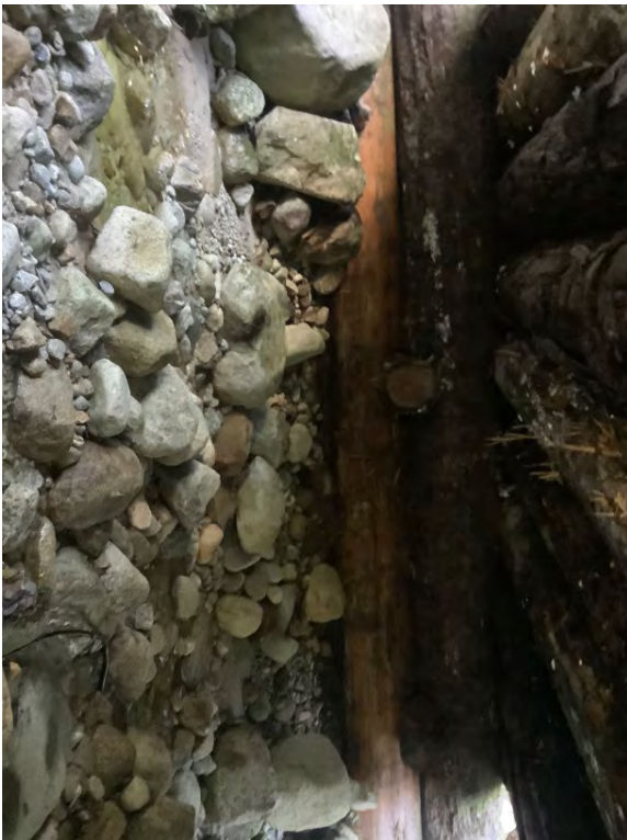
Left Bank Abutment when facing downstream
